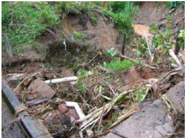
De ravage na de overstroming.
